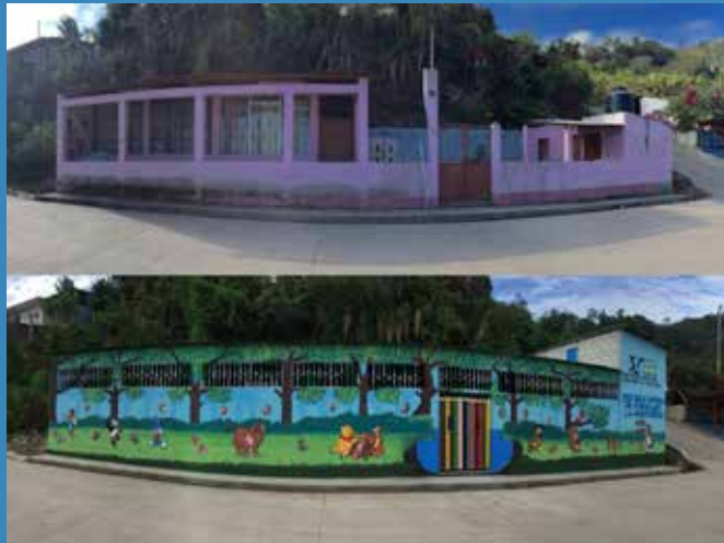
La Montañita nursery, before and after reconstruction.
